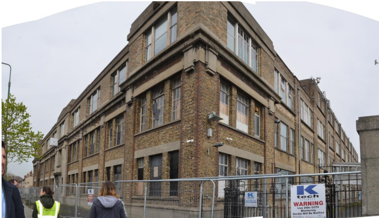
FIGURE 14.20: OBLIQUE VIEW ALONG SOUTHERN (FRONT) AND EASTERN ELEVATION OF BLOCK A.
