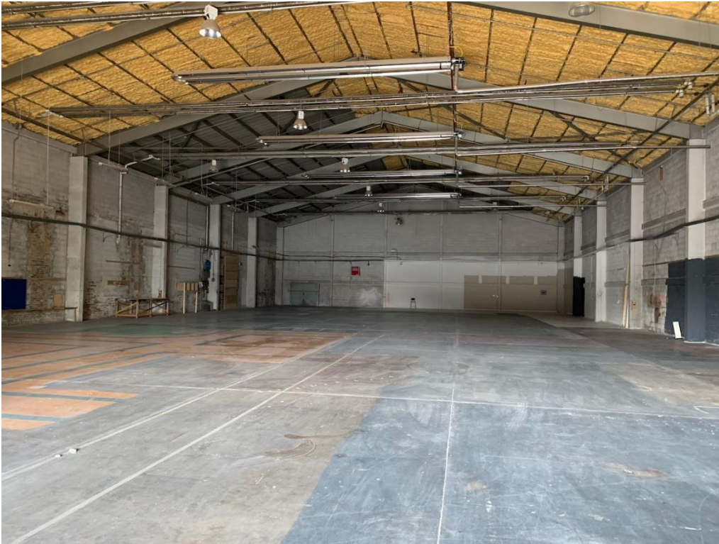
Plate 10.5: Internal view of one of the buildings to be demolished.
