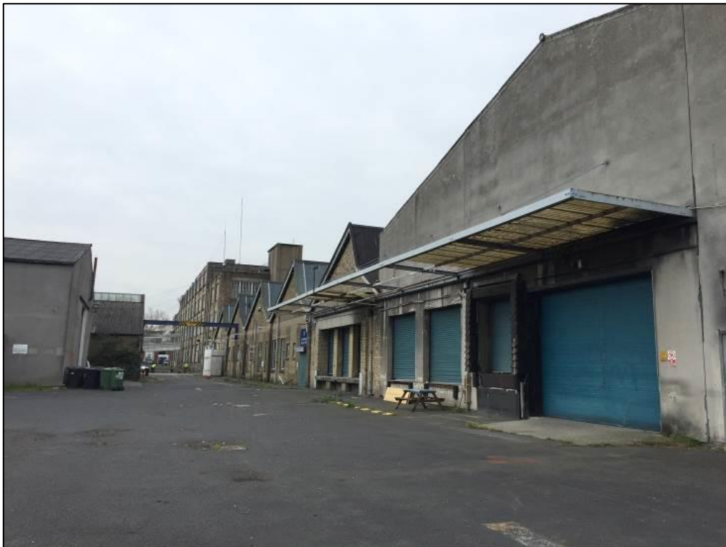
PLATE 13.4 ENTRANCE TO THE SITE, FACING NORTH
