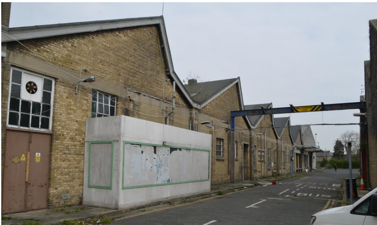
FIGURE 14.23: OBLIQUE VIEW ALONG THE EASTERN ELEVATION OF BLOCK B, LOOKING NORTH TOWARDS THE LATER EXTENSION.
