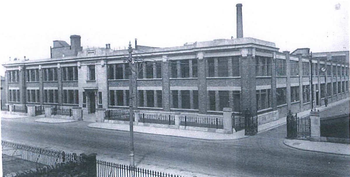
FIGURE 14.10: UNDATED PHOTOGRAPH OF THE FRONT FAÇADE ALONG SOUTH CIRCULAR ROAD, SHOWING THE SOUTH AND EAST ELEVATIONS IN THE MID-LATE 1920S. THIS PHOTOGRAPH PRE-DATES THE C. 1929 ADDITION OF THE SECOND FLOOR.
